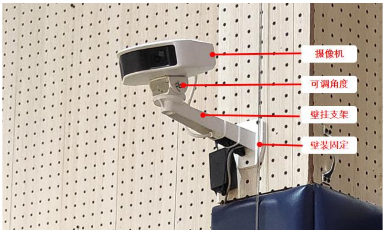
Figure 4-3 Fixed Wall Mount Installation
